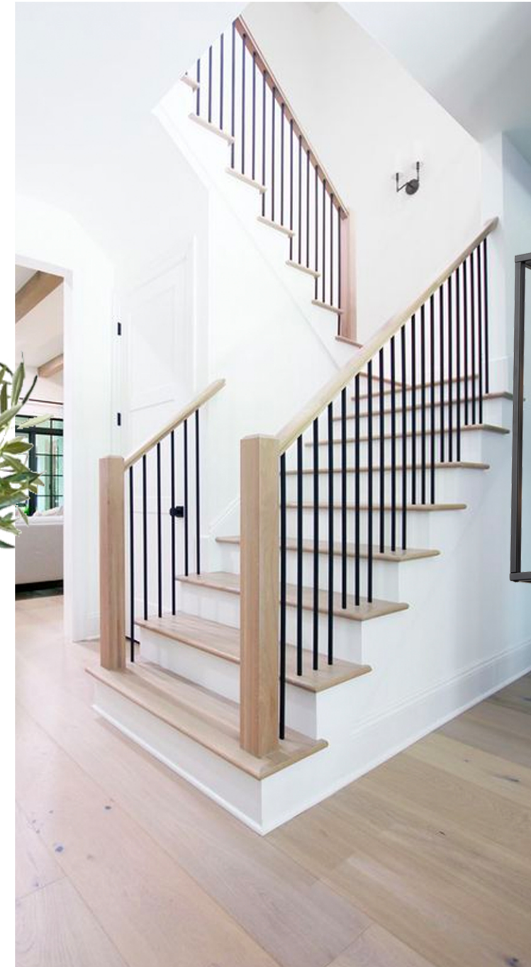
Piano treatment staircase with straight iron pickets and oak handrails
